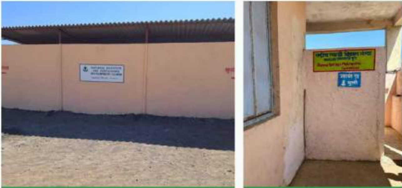
Figure 28: Toilet renovated in Government School, Karanjale (left) Taleran (right)
